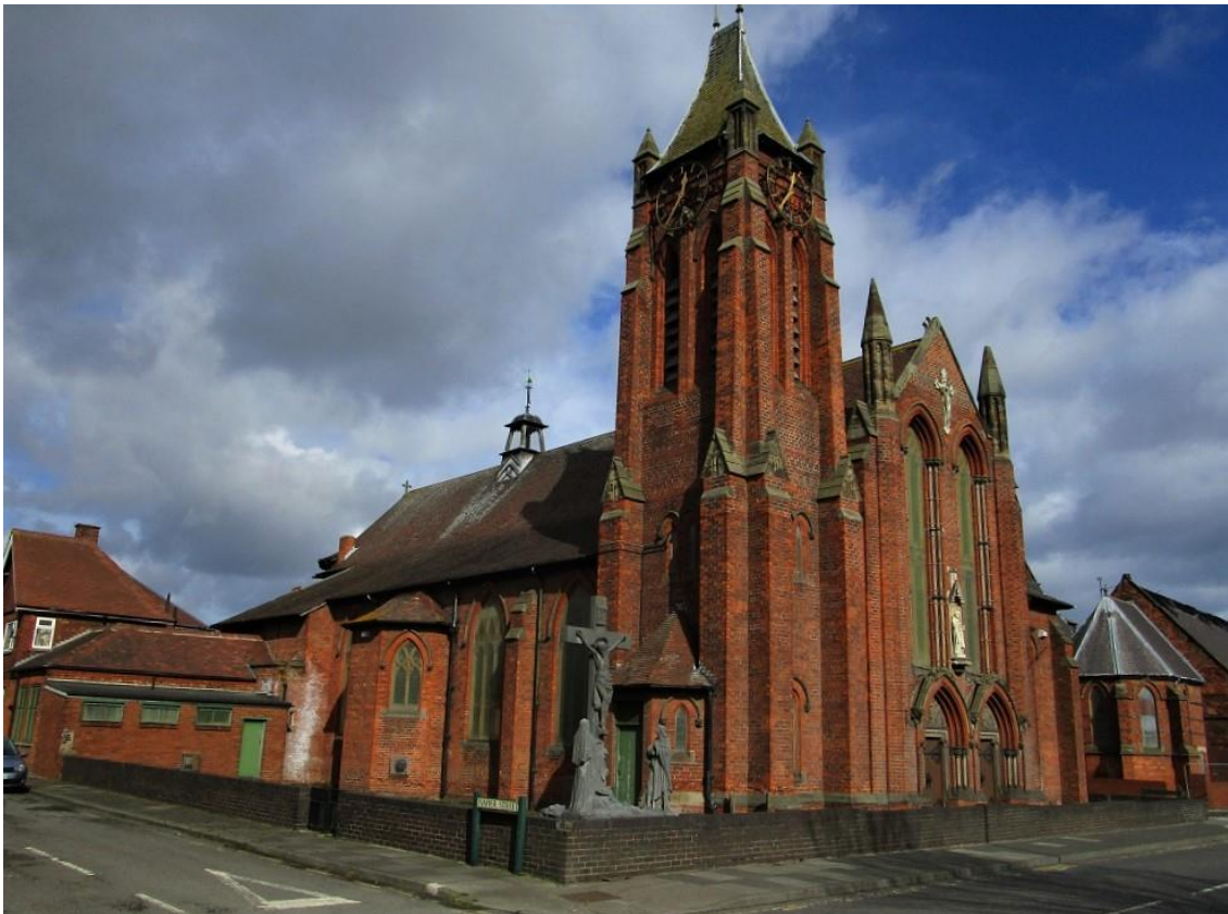
Fig. 20: View from northwest
