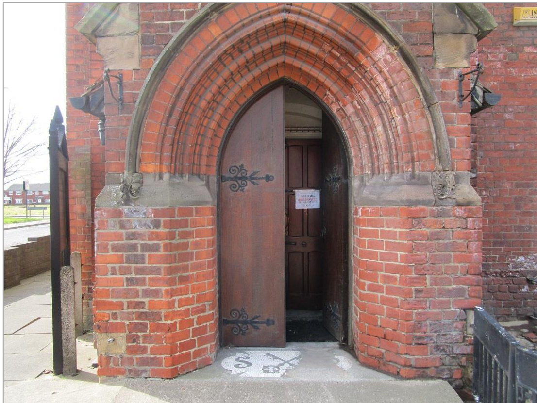
Fig. 25: South porch, with worn cross keys mosaic at threshold
