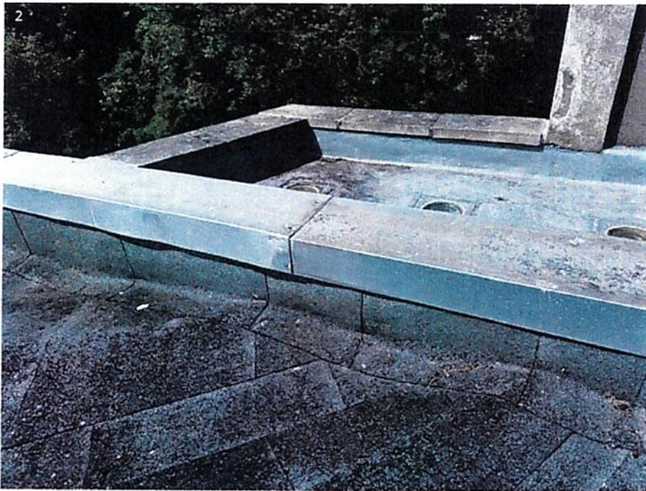
Existing parapet capping to be removed and boarded over with plywood
