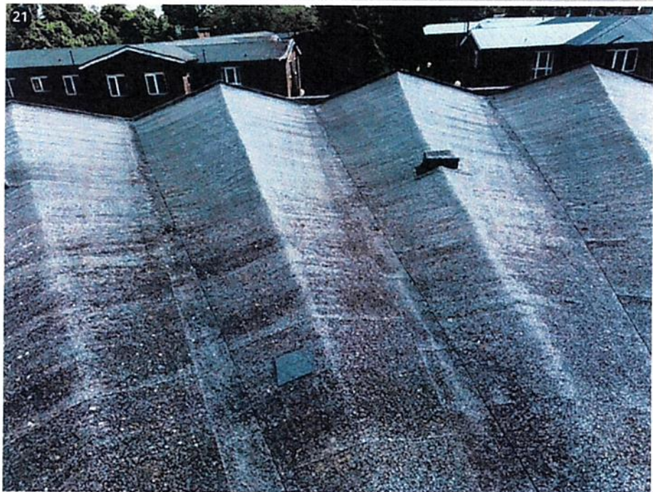
Existing membrane showing signs of mineral loss and deterioration
