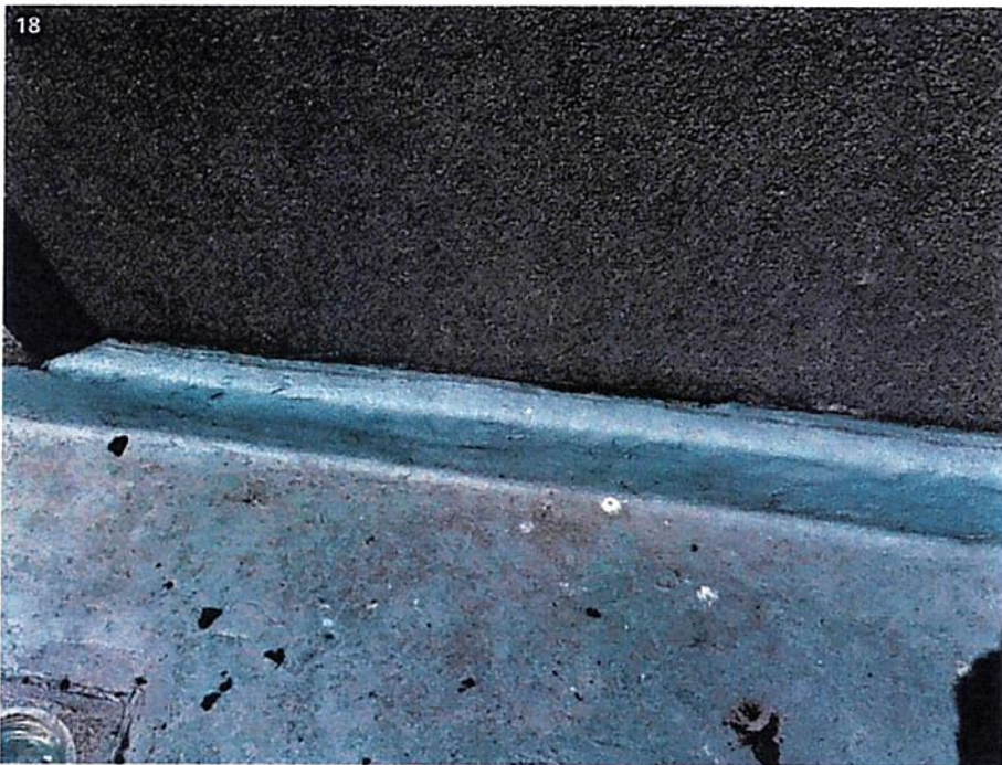
Poor upstand detail
