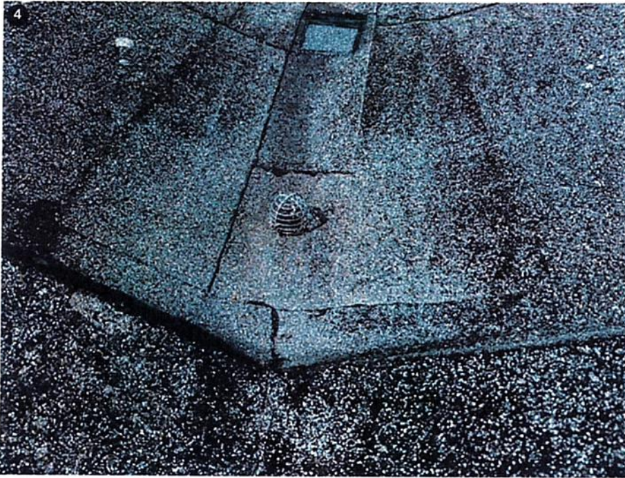
Core to gutter area showed no insulation
