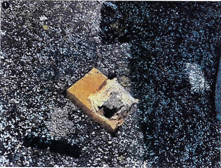
Core sample taken revealed fibreboard insulation 25mm R1
