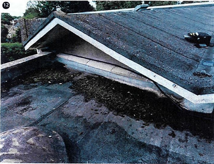
Area of moss growth indicating ponding water
