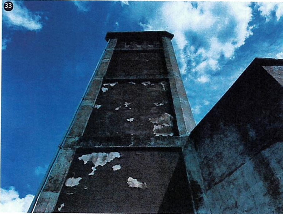
Existing condition of tower - This could be cladded to encapsulate or treated
