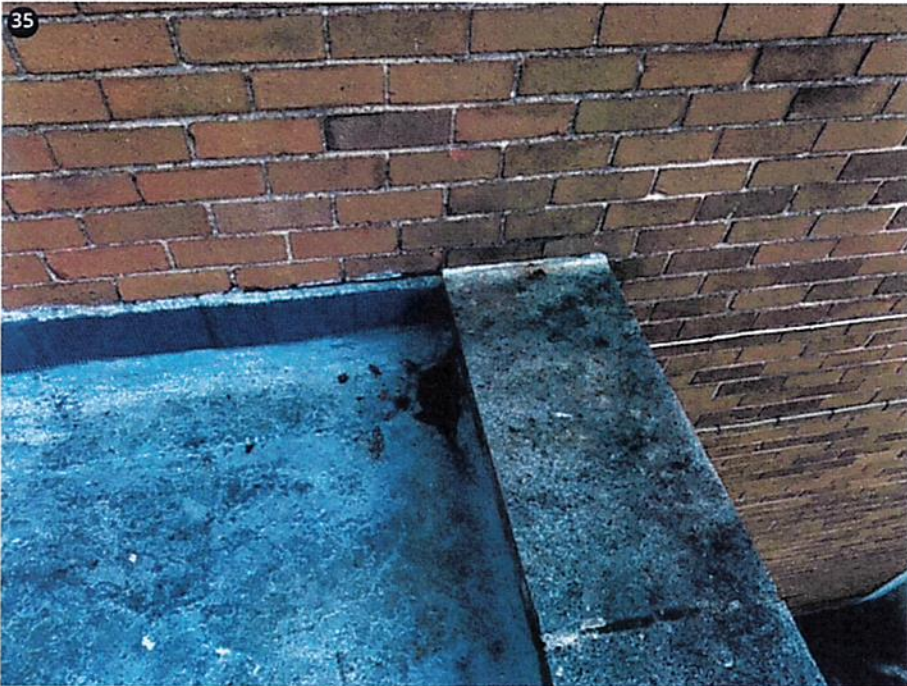
Poor detailing noted to upstands
