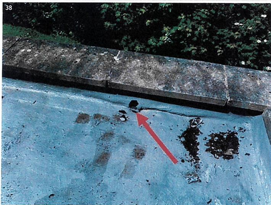
Failed section to parapet
