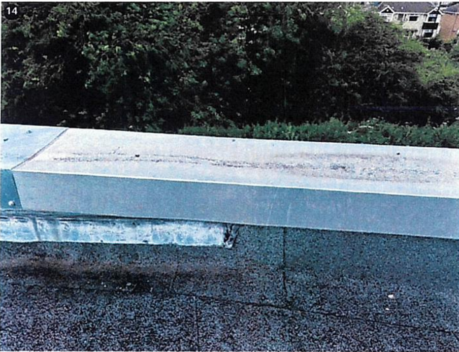
Previous repairs have been carried out
