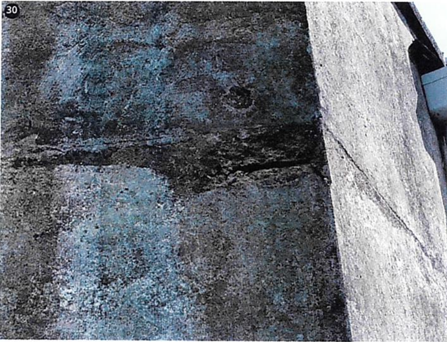
Spalling to vertical section
