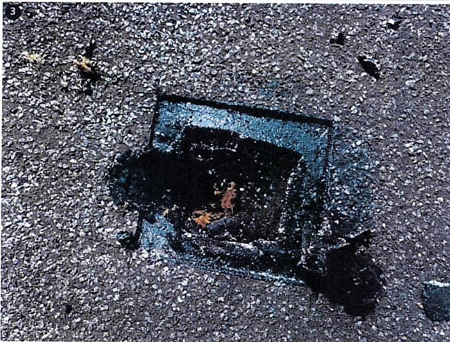
Core sample to R2 showed saturated insulation over concrete deck
